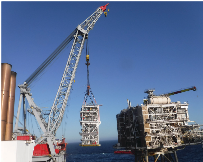
Positioning the 800 tonne topside module
